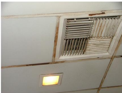
The appearance of a ceiling can be improved immensely by cleaning the tiles, covering rusted & stained metal t-bars, and replacing rusted vents. Routine cleaning of ceilings can improve its appearance 70-80% without damage overnight and prolong its life.
